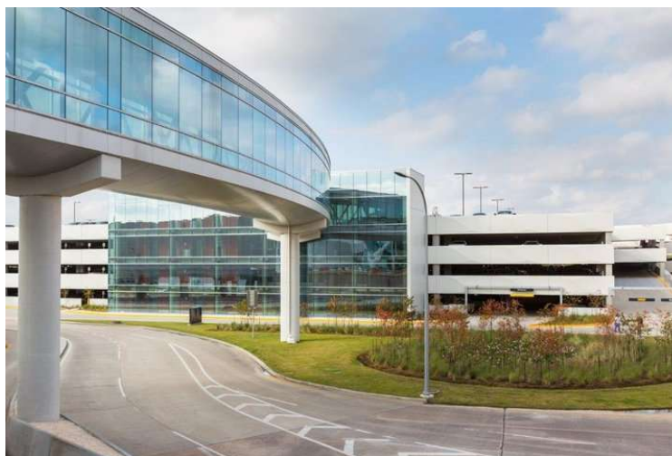
Blue Parking Garage
