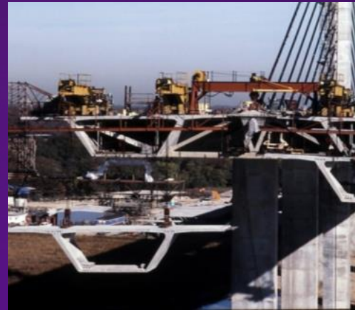
B&W lift of Segment Over Shipping Channel, Richmond Va.
