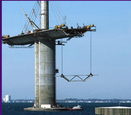
B&W lift of Segment Over Shipping Channel, Tampa Florida
